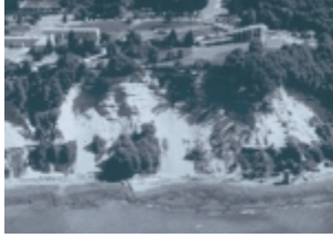
Buildings near unstable cliff of Ice Age sand and silt, U.B.C. University of B.C.
